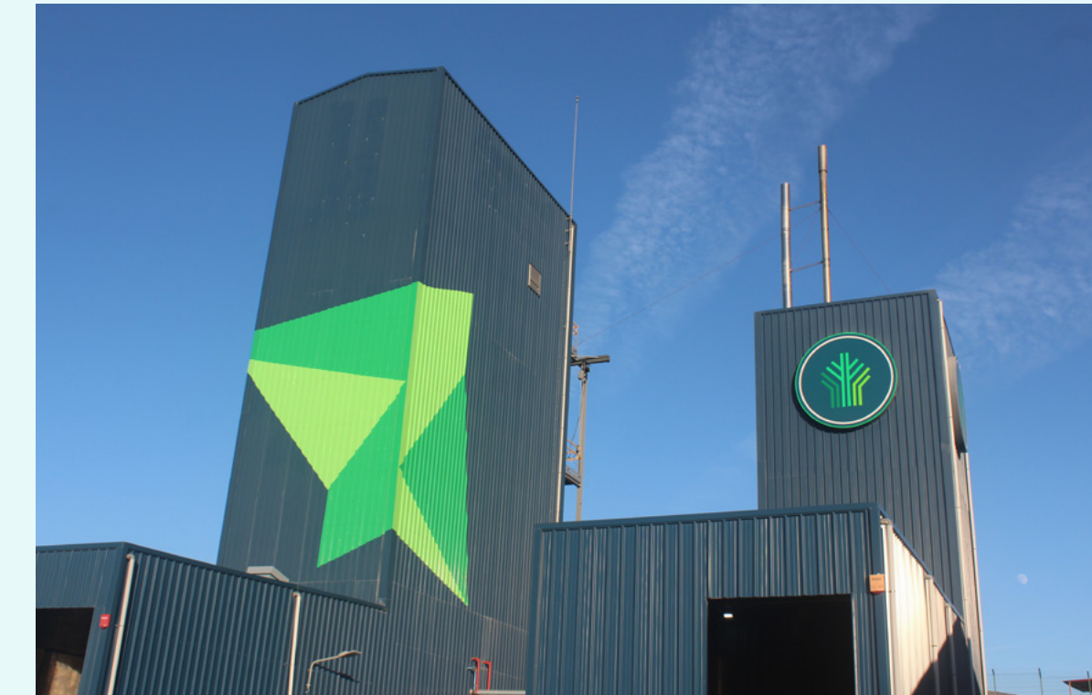
Drying tower at Ascenza industrial plant, in Setúbal, Portugal
