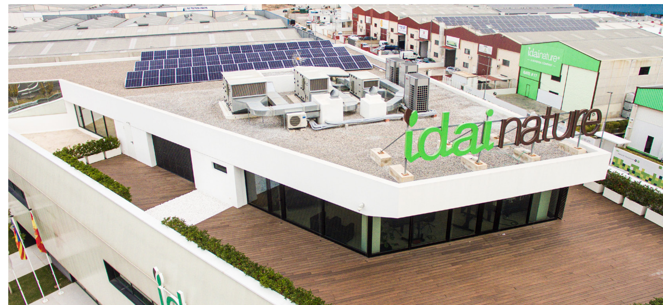
Photovoltaic panels on our site in Valencia, Spain
